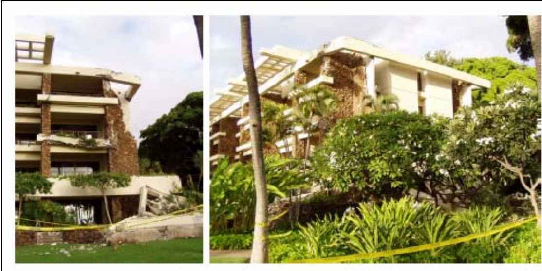
Figure 42 Collapse of concrete trellis frame at Mauna Kea Beach Hotel. (Photograph courtesy of Ian Robertson)
