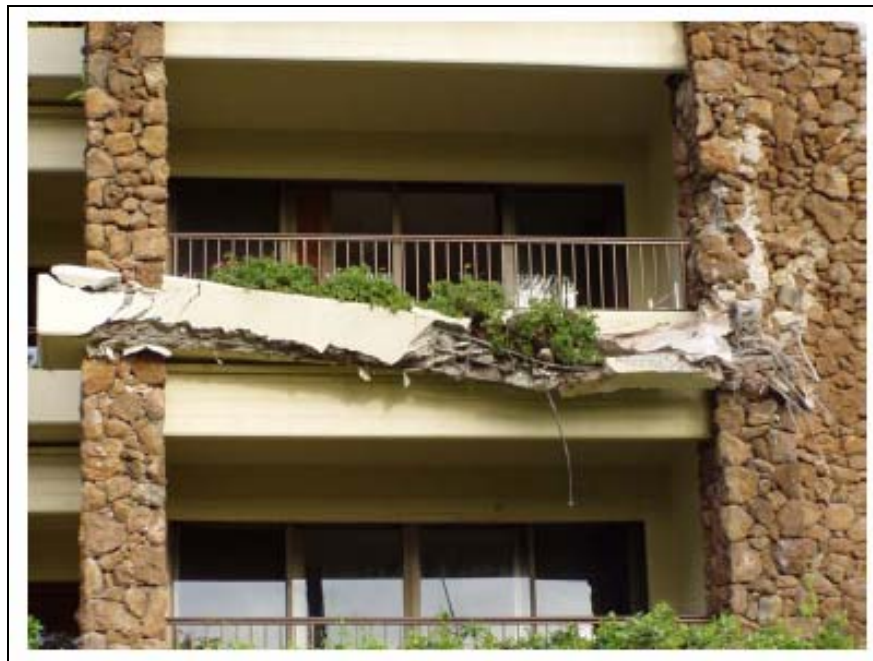
Figure 43 Damage to balcony due to impact from falling debris (Photograph courtesy of Ian Robertson)
