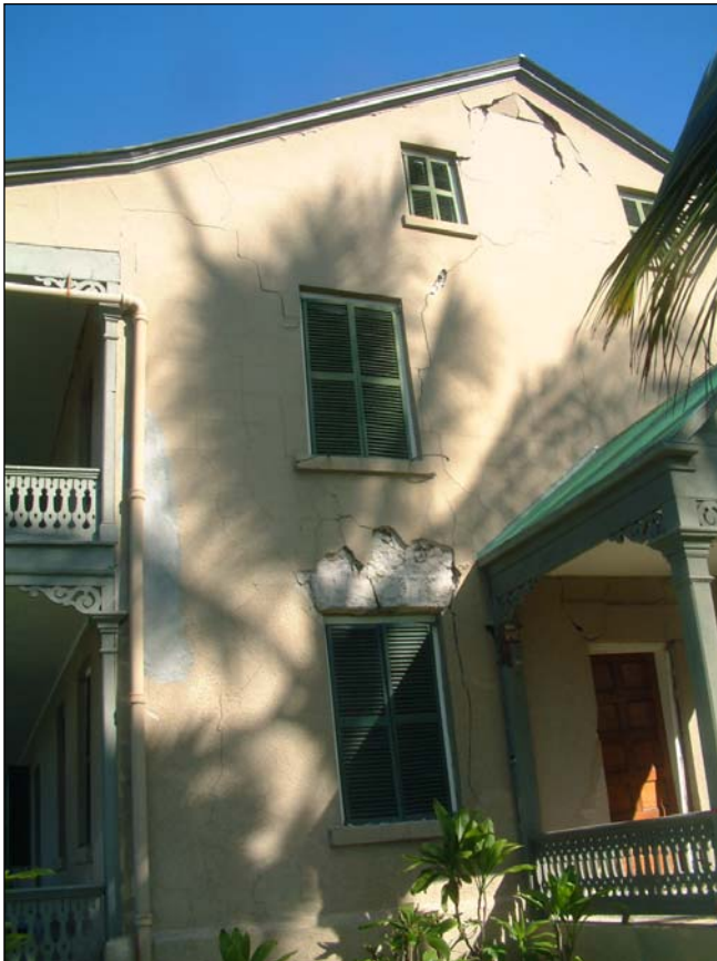
Figure 29 Damage to the plaster finish and masonry of a gable end wall of Hulihe‘e Palace
