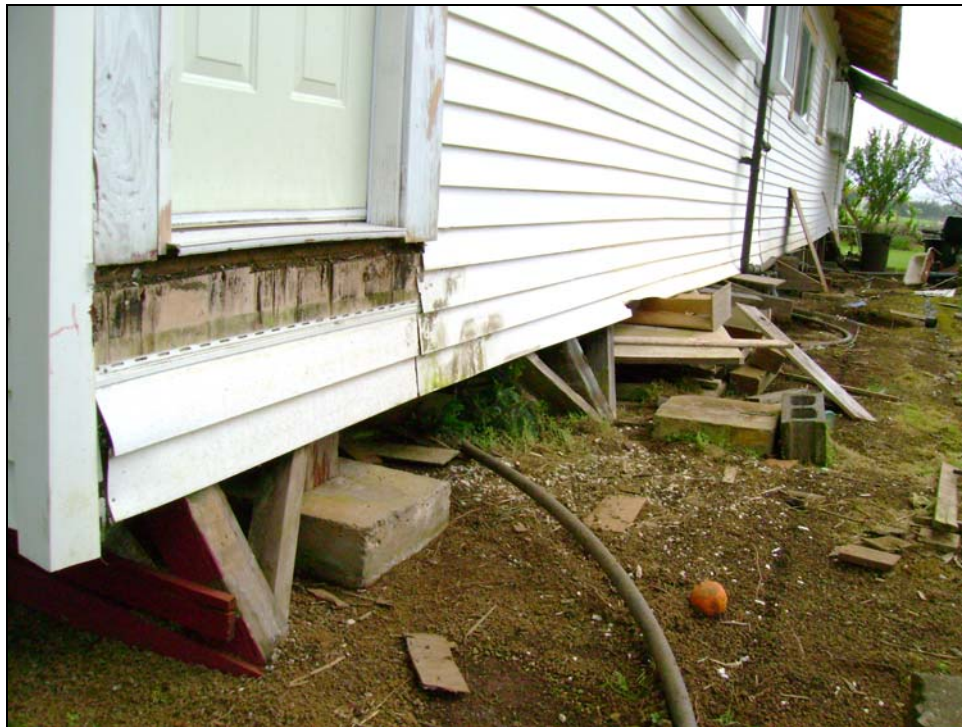
Figure 36 Collapse of the Post and Piers of a Single Wall Home; note lateral displacement from footing (Photograph courtesy of Clifford Lau)
