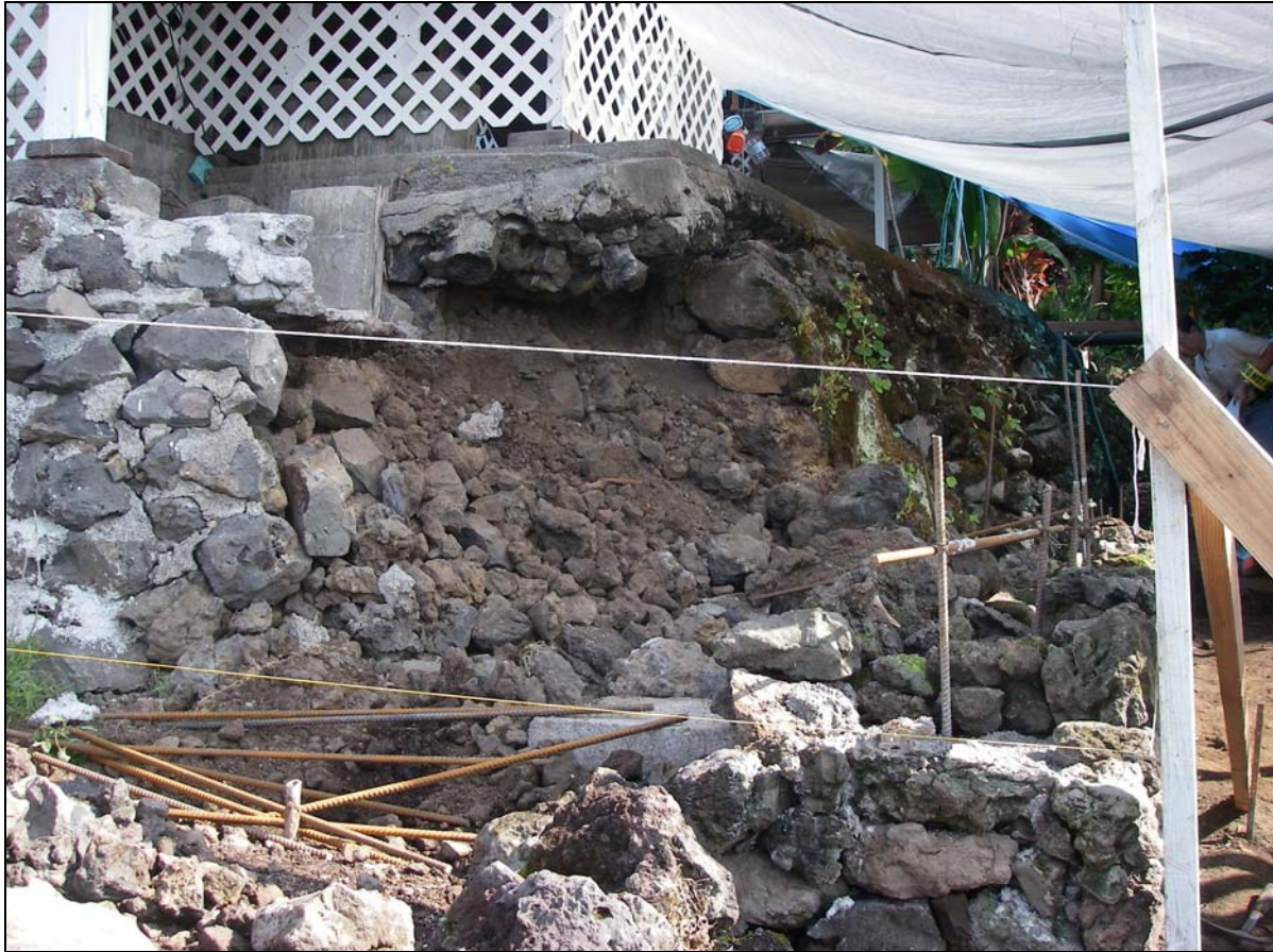
Figure 38 Failure of a loosely fitted and mortared lava rock wall causing undermining of single family home; note the beginning of a replacement wall construction in foreground (Photograph courtesy of Glenn Miyasato)
