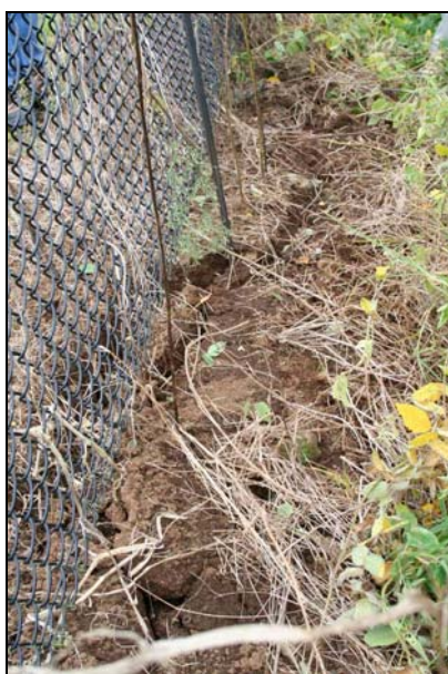
Figure 17 Cracking and stability failures on the crest of reservoir dams
