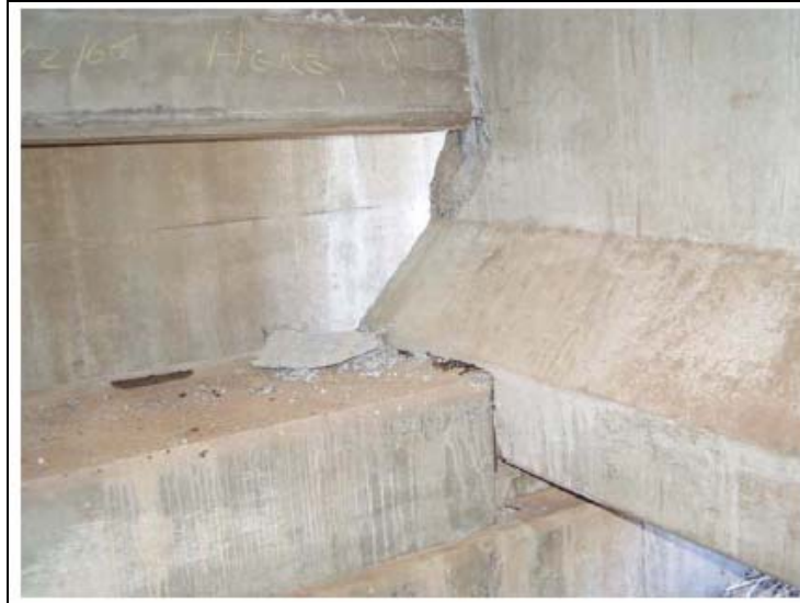
Figure 23 Damage to web of AASHTO girder at Abutments (Photograph courtesy of Ian Robertson)
