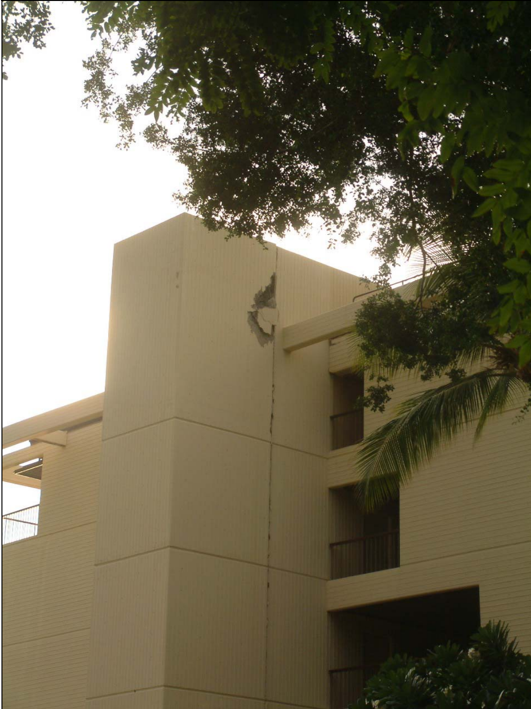
Figure 45 Damage to concrete exhaust flume at connector plate – east side. (Photograph by Gary Chock)
