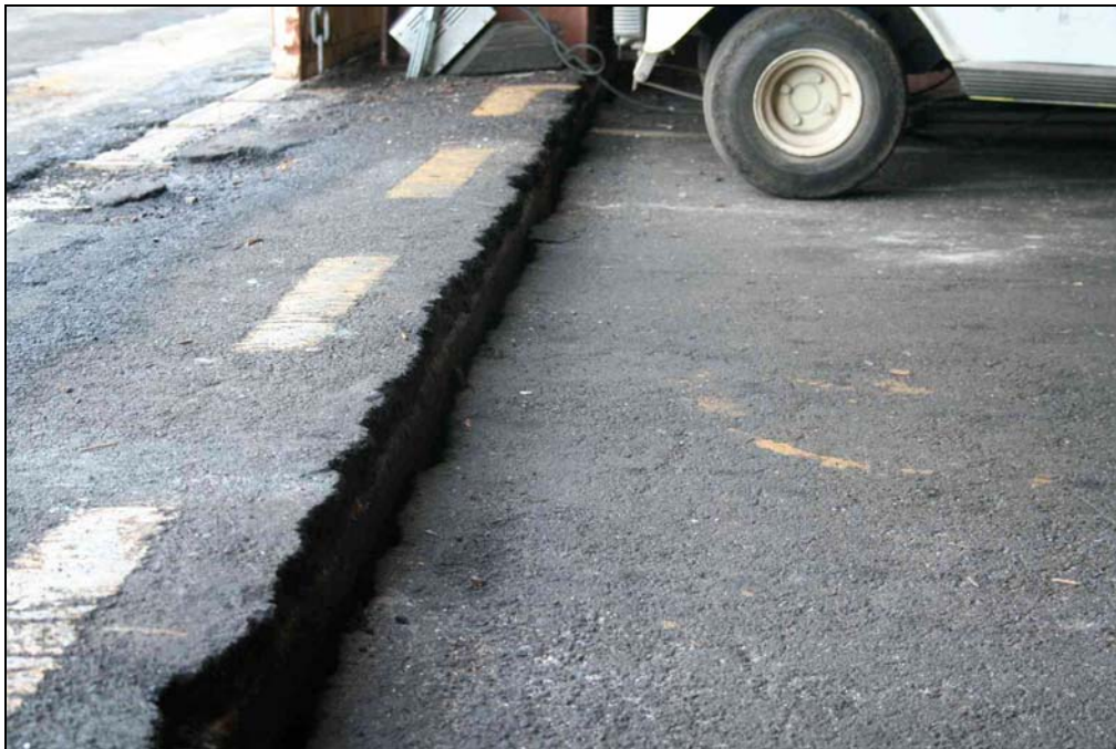
Figure 20 Liquefaction induced lateral and vertical displacements of approximately 6 inches at port facility, Kawaihae Harbor (Photograph by Peter Nicholson)
