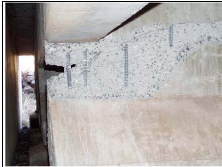
Figure 24 Shear key and bridging beam between AASHTO bridge girders (Photograph courtesy of Ian Robertson)
