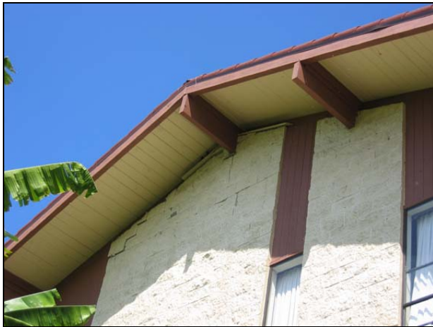
Figure 47 Out-of Plane Shear failures at the gable end CMU walls, Paniolo Club, Waikoloa Village (Photographs courtesy of Jeffrey Hanyu)
