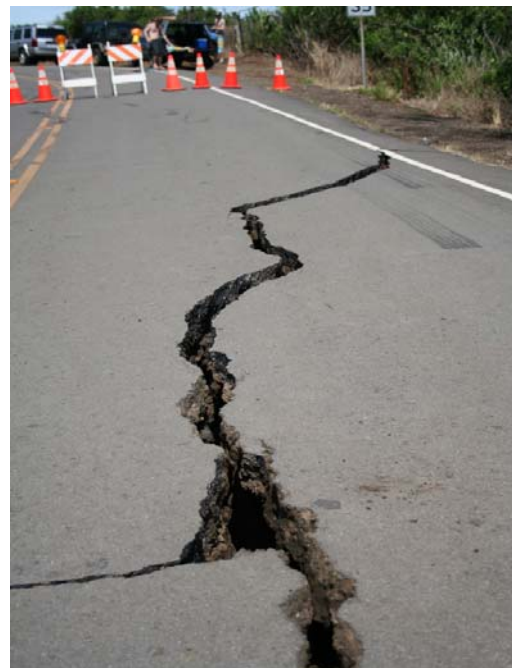
Figure 11 Highway Embankment and Roadway Failures
