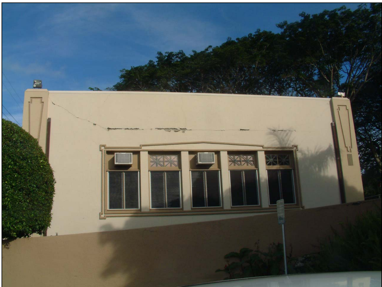
Figure 50 Horizontal and diagonal cracks in concrete walls of Bank of Hawaii in Kapaau, near Hawi (Photograph by Gary Chock)
