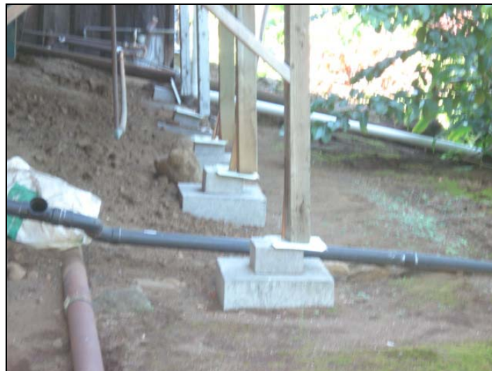
Figure 31 Tall unanchored posts on the verge of slipping off their foundation piers; note splitting of wood columns at their bases (Photograph courtesy of Kylie Yamatsuka)
