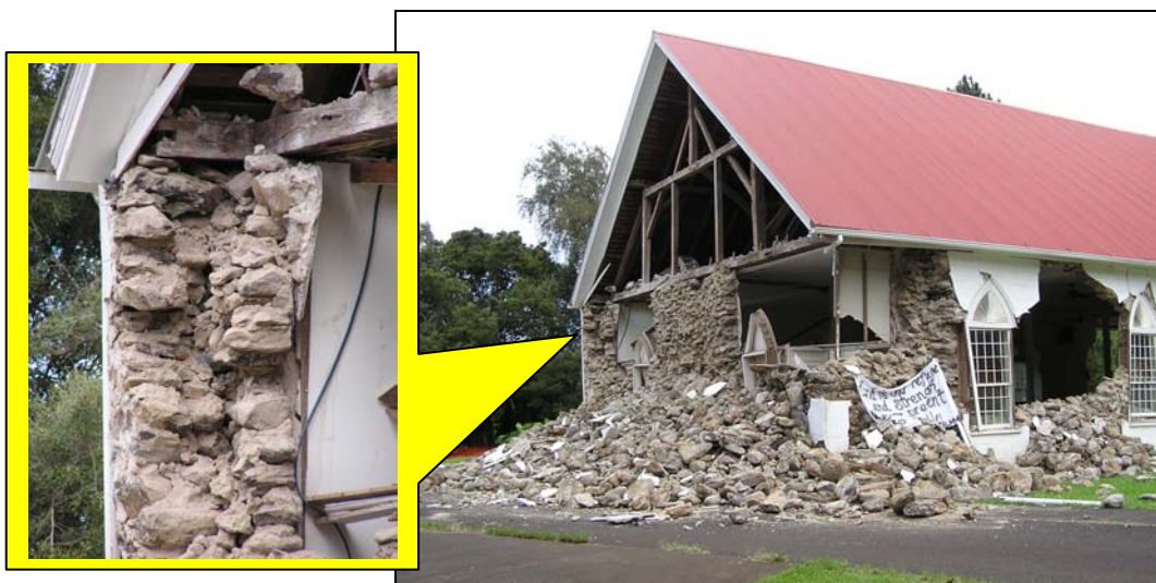
Figure 28 Unreinforced basalt rock-masonry walls filled with low strength mortar and smaller rubble (Photograph courtesy of Edward Medley)
