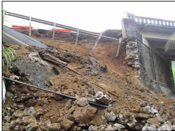
Figure 12 Failure of Bridge Approach Embankment On Highway 19 Due to a Retaining Wall Collapse (Photographs courtesy of State of Hawaii Dept of Transportation, Highways Division, and Hawaii County Civil Defense Agency)
