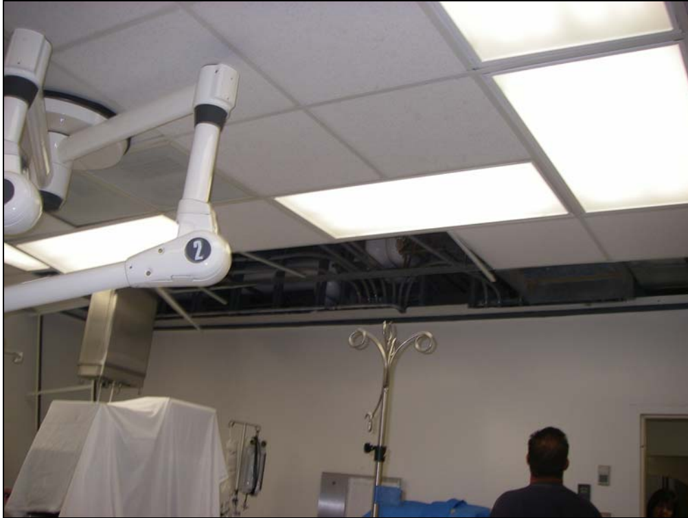
Figure 51 Fallen Ceiling in the Operating Room, Kona Community Hospital (Photograph courtesy of Glenn Miyasato)
