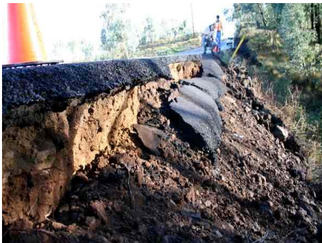
Figure 11 Highway Embankment and Roadway Failures
