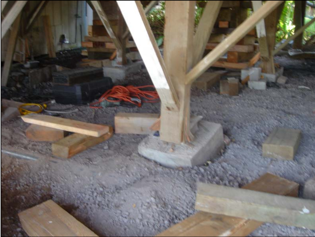
Figure 33 Splitting of a Post Base with Lateral Displacement (Photograph courtesy of Ron Iwamoto)
