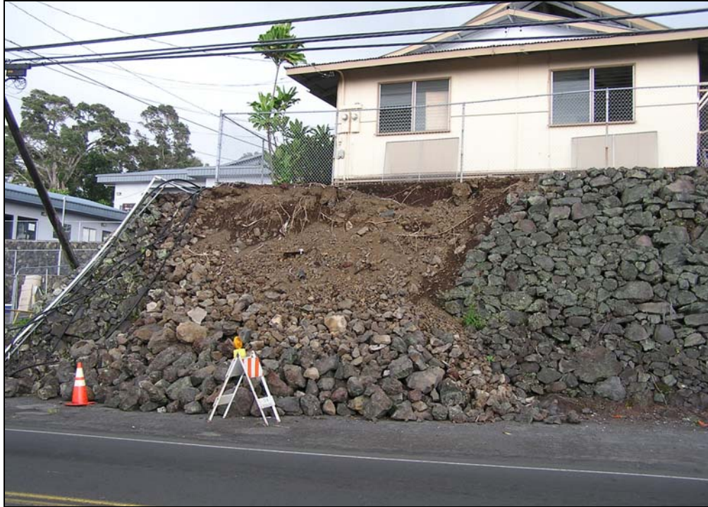
Figure 39 Failed stacked rock retaining wall in Captain Cook, adjacent Hwy 11. (Photograph courtesy of Edward Medley)
