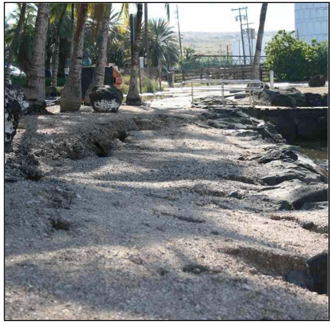
Figure 19 Examples of sand boils and lateral spreading, Kawaihae Harbor (Photographs courtesy of Peter Nicholson)
