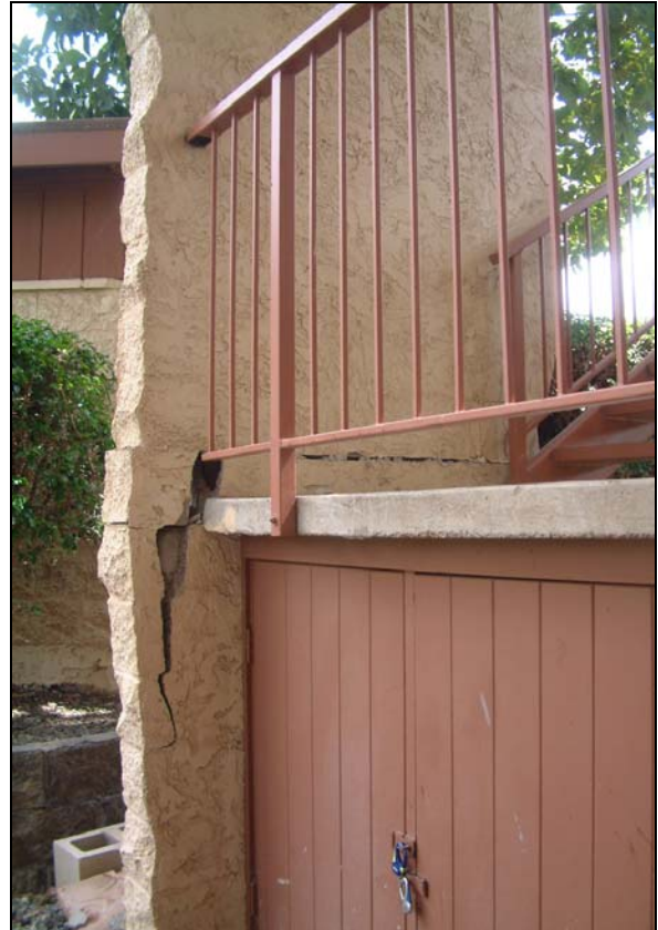
Figure 49 Exit Stair Support Wall with Spalled End Cells and Lateral Displacement In-Plane and Out-of-Plane (Photograph by Gary Chock)
