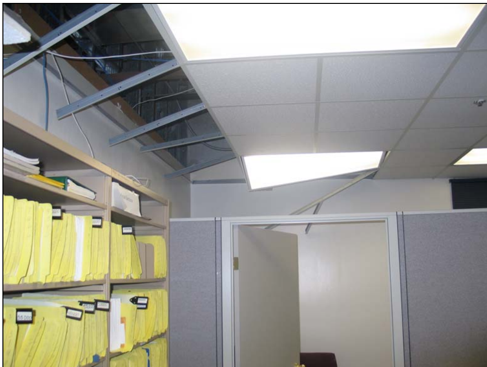
Figure 52 Ceiling Damage in a Medical Records Room at Kona Community Hospital (Photograph courtesy of William Holmes)
