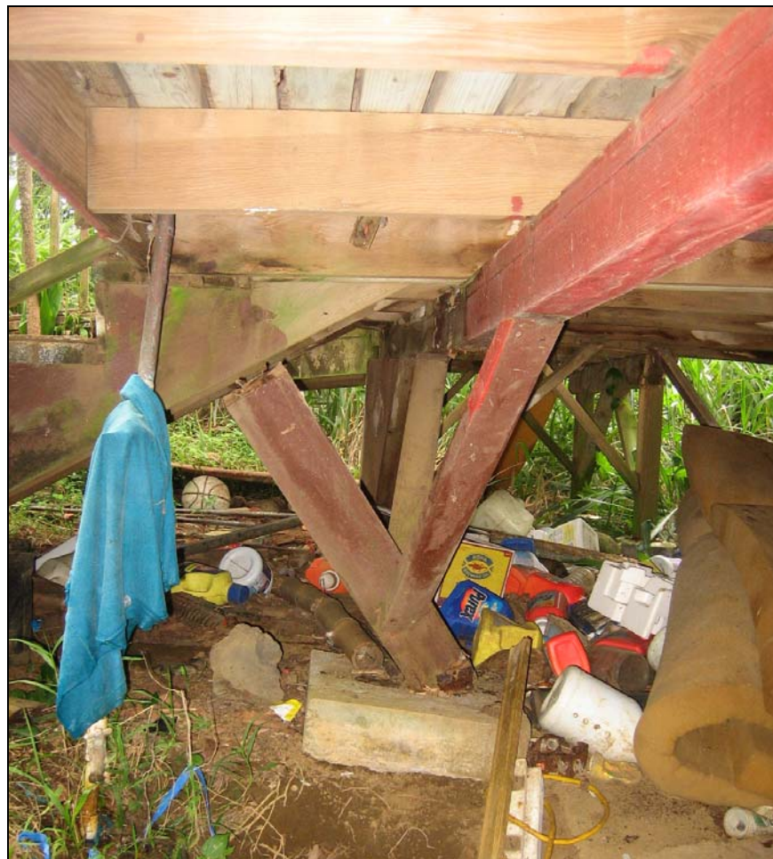
Figure 32 Detachment of a Post at the Top and Bottom at a Sloping Hillside Site (Photograph courtesy of Tim Waite)
