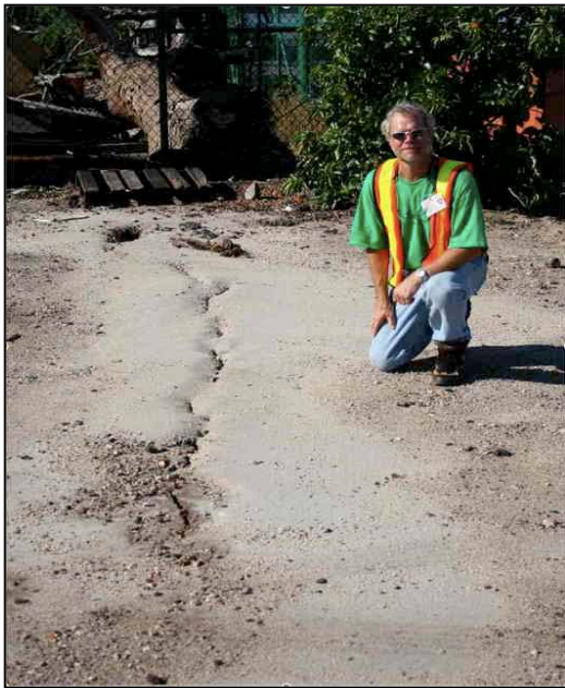
Figure 19 Examples of sand boils and lateral spreading, Kawaihae Harbor (Photographs courtesy of Peter Nicholson)
