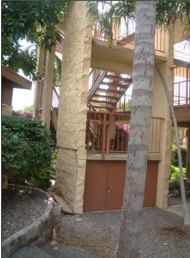
Figure 49 Exit Stair Support Wall with Spalled End Cells and Lateral Displacement In-Plane and Out-of-Plane (Photograph by Gary Chock)
