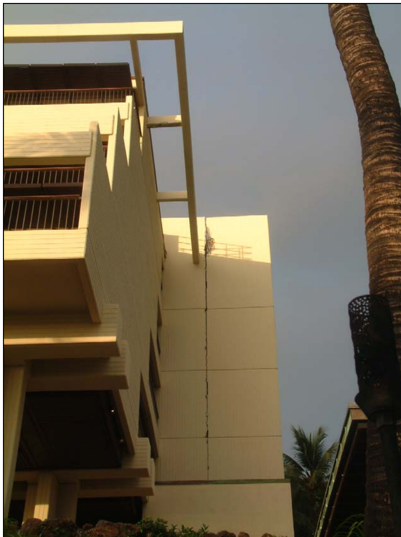
Figure 44 Damage to concrete exhaust flume at connector plate – west side. (Photograph by Gary Chock)
