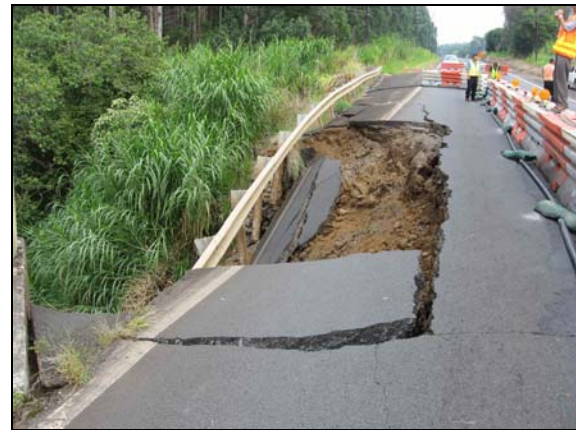
Figure 12 Failure of Bridge Approach Embankment On Highway 19 Due to a Retaining Wall Collapse (Photographs courtesy of State of Hawaii Dept of Transportation, Highways Division, and Hawaii County Civil Defense Agency)
