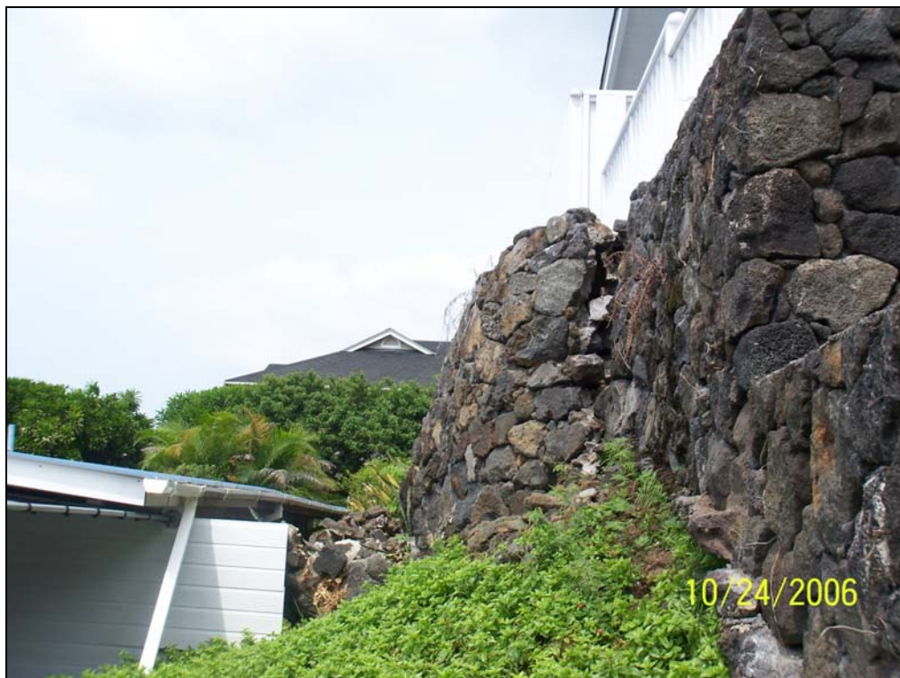
Figure 40 Failure of a dry-stacked lava rock wall threatening a neighboring property (also note damaged carport) (Photograph courtesy of Lee Takushi)
