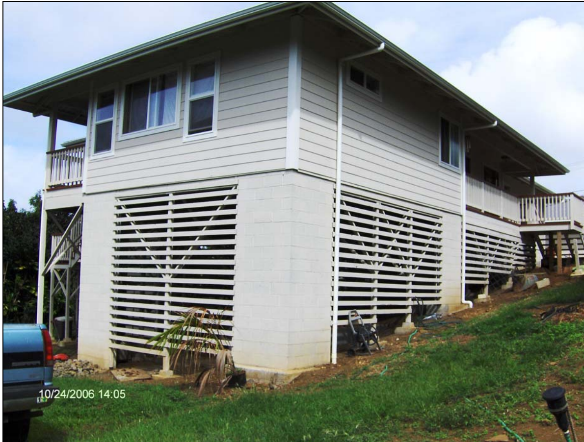
Figure 37 An example of an undamaged home with an improved form of elevated floor framing on a hillside utilizing masonry corner walls (Photograph courtesy of Gary Suzuki)
