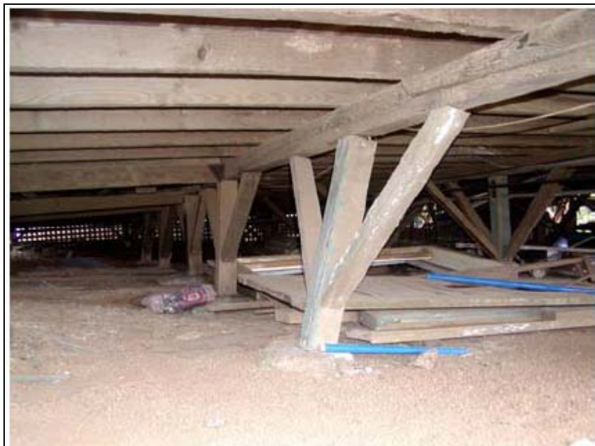
Figure 34 Rotational Instability Mode of Post and Pier "Single" Wall Homes (Photograph courtesy of Ian Robertson)
