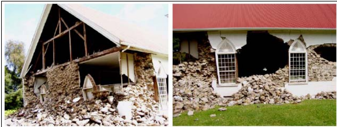
Figure 27 Roof trusses supported by interior columns and window frames after wall collapse . (Photographs courtesy of Ian Robertson)
