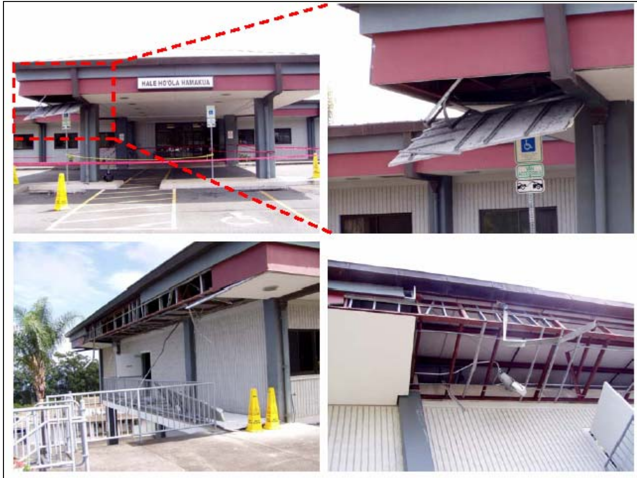
Figure 53 Damage to exterior stucco ceilings at Hale Ho'ola Hamakua medical facility in Honoka'a (Photographs courtesy of Ian Robertson)
