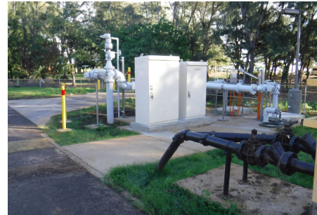
Wailua upgraded pump station site
