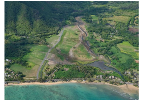
Punaluu Stream Restoration Project at Substantial Completion
