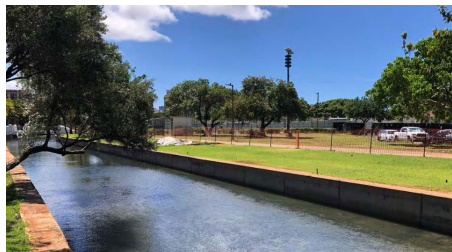
Ala Moana Regional Park Improvements. The collapsed wall on far side of the existing canal was replaced with mechanically stabilized earth wall with geosynthetic reinforcement.
