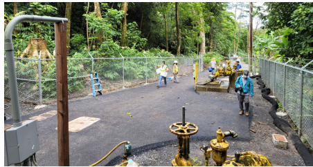
Waihole Well Site Repaired
